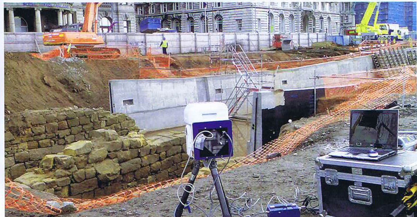
Canal project Liverpool, England
